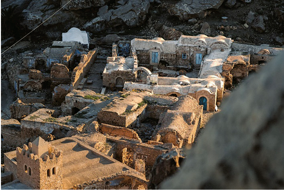
Figure 10: Vaulted roofs of the dwellings in Zriba Olia village.
