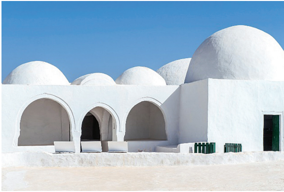
Figure 15: A mosque in Djerba whitewashed with lime plaster.
