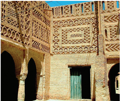
Figure 13: The brick cladding in houses facades in Tozeur and Nafta cities.
