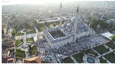
Şl. 2: Fatih Külliyesi ( https://rayhaber.com/2020/07/fatih-camii-ve-kulliyesi-hakkinda/fatih-camii-ve-kulliyesi-hakkinda/ ).
