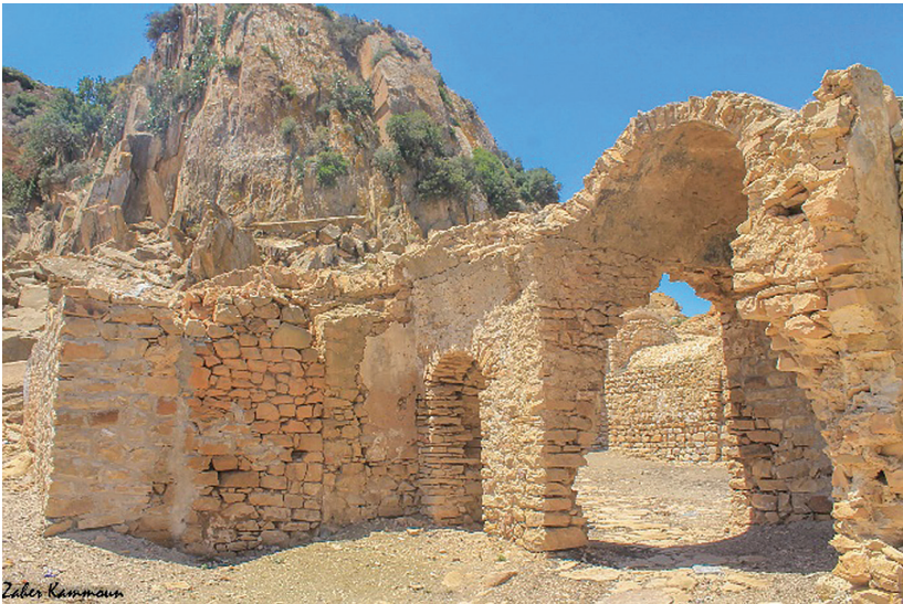
Figure 9: A picture showing the wall thickness in a dwelling in Zriba Olia village.
